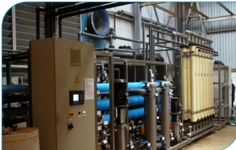
Figure 5: Example of a possible technology train for the demineralisation step in the MinWaterCSP water management.
