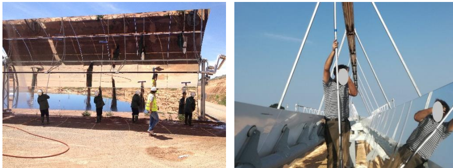
Picture 1&2: Manual cleaning of mirrors consumes a large amount of water (© ECILIMP and Soltigua)
