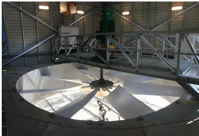
Figure 4: Installed CSP fan (© Kelvion Thermal Solutions (Pty) Ltd and ENEXIO Management GmbH)
